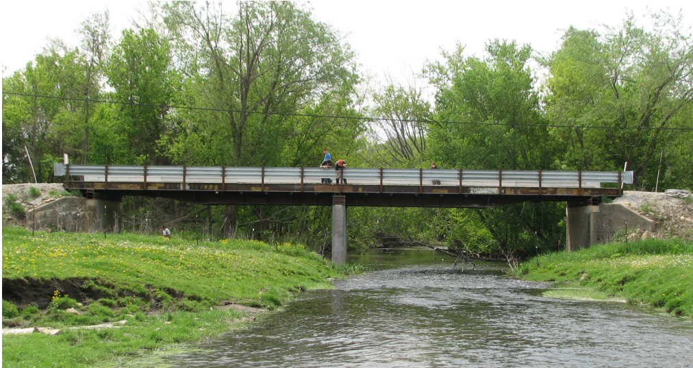
Figure 2.4. Completed Buchanan County RRFC Bridge 4 (BCB4).
