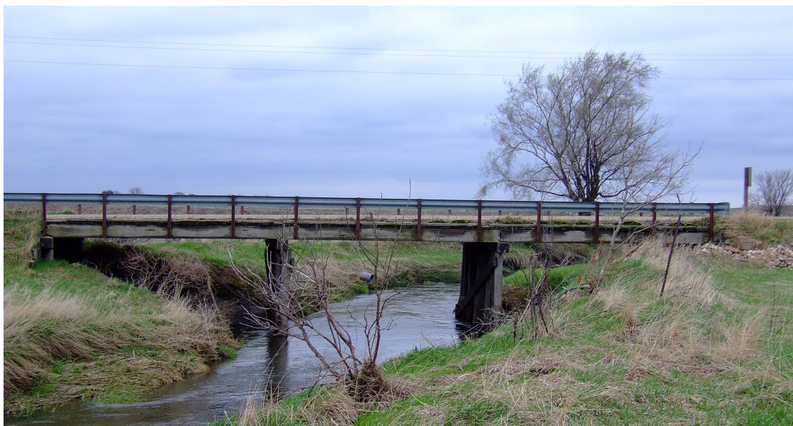
Figure 4.2. Previous bridge at WCB3 site.
