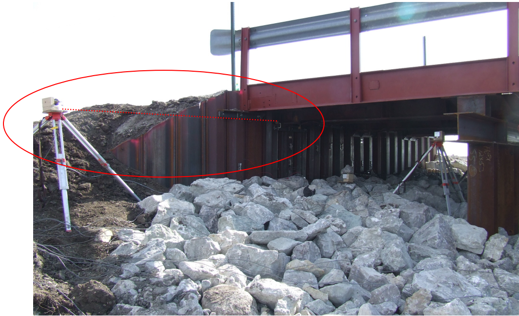
Figure A.11. Instrumentation measuring displacement perpendicular to traffic.
