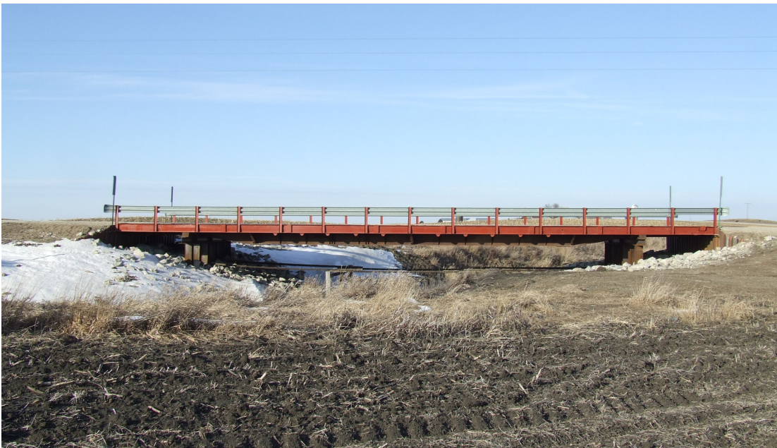
Figure A.1. Winnebago County RRFC Bridge 3 (WCB3).
