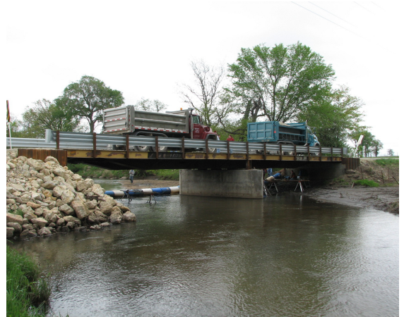
a. Side view of two-truck load test
