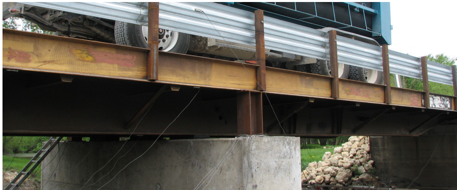
b. I-shaped Support at Exterior Girder
