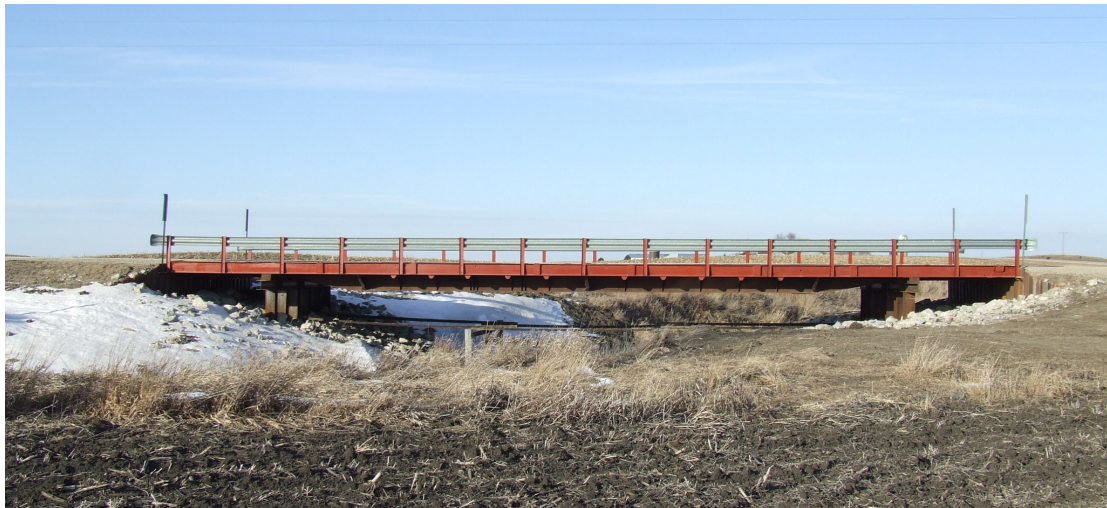
Figure 4.5. Completed Winnebago County RRFC Bridge 3 (WCB3).
