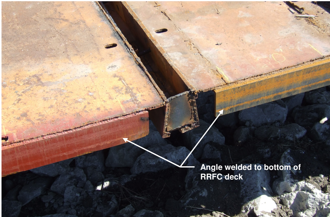
Figure A.7. Angle welded to bottom of RRFC deck.
