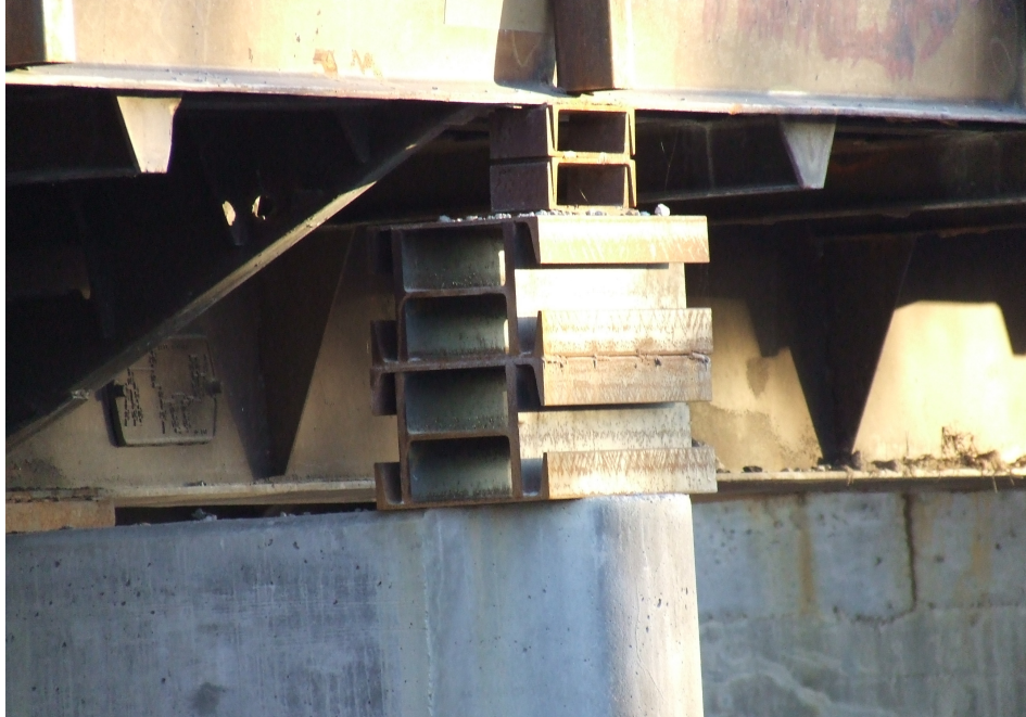
Figure 2.3. Miscellaneous I-shapes used as exterior girder support.
