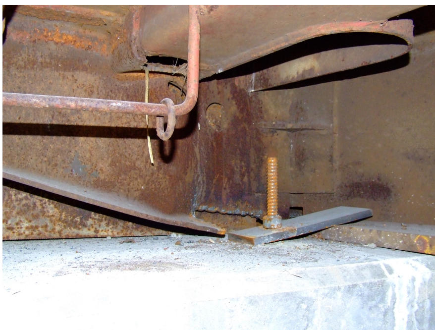
Figure 3.3. Clip angle to attach RRFC to abutment.
