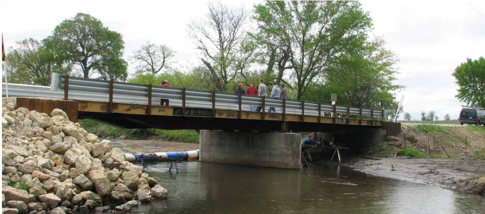
Figure 3.6. Completed Buchanan County RRFC Bridge 5 (BCB5).
