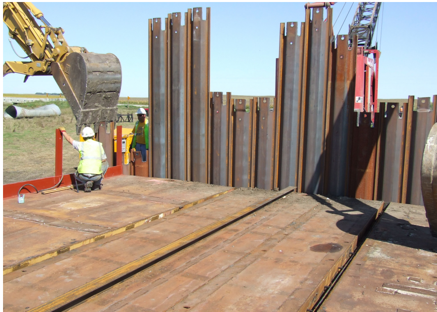
Figure A.6. East abutment after driving.
