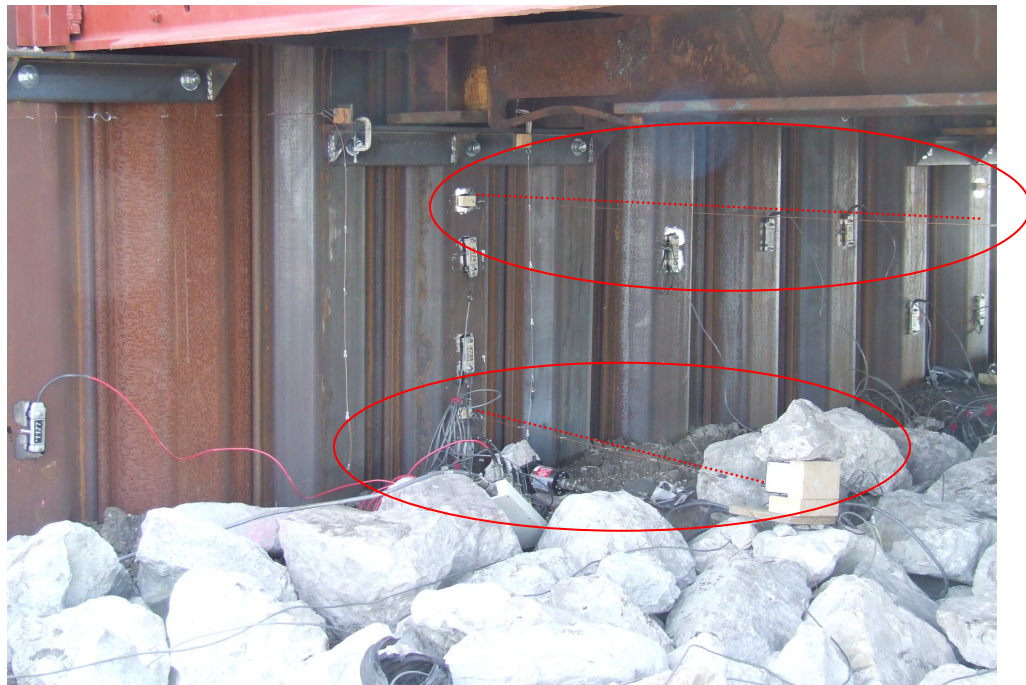
Figure A.12. Instrumentation measuring displacement in the direction of the bridge.
